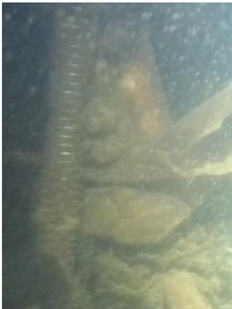
Figure 17 : Trash on the pipe
