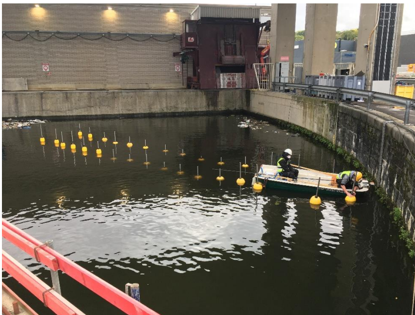
Figure 12: PROCOM are correcting the height of the buoys
