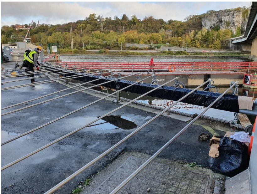
Figure 10 : the first barrier ready to be launch
